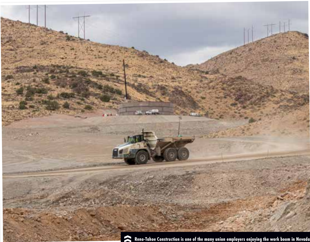
Reno-Tahoe Construction is one of the many union employers enjoying the work boom in Nevada.
