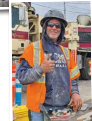
Billy Conrad is pumping concrete at the SFPUC building.
