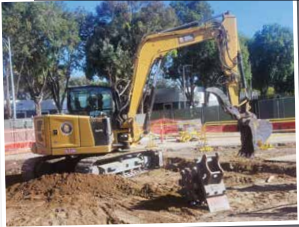
>> Excavator Operator Jeffrey Jones backfills for the Equinix Data Center.
