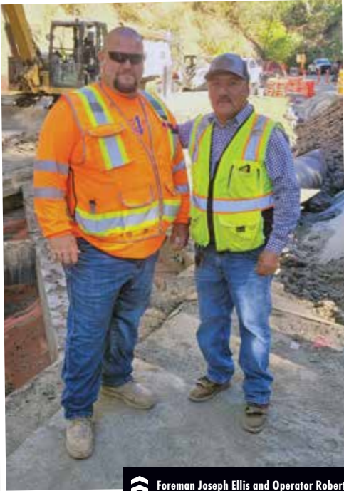
Foreman Joseph Ellis and Operator Roberto Ruiz work at the Morgan Territory Road Bridge Replacement project.
