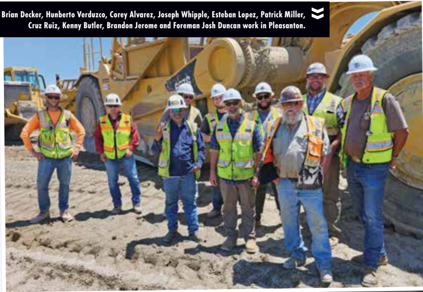
Members work on the planned development at the old Kaiser Rock Quarry.
