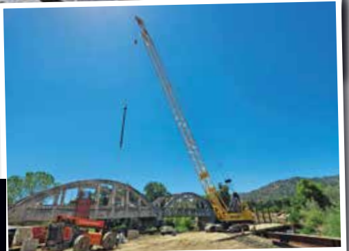
Members with Steelhead Constructors work at the Rumsey Bridge Replacement project.
