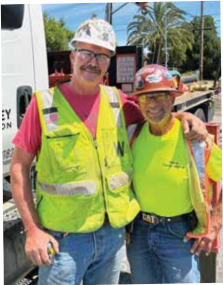
Greg Woolworth and Murray S. Weber are installing new water infrastructure. >>
