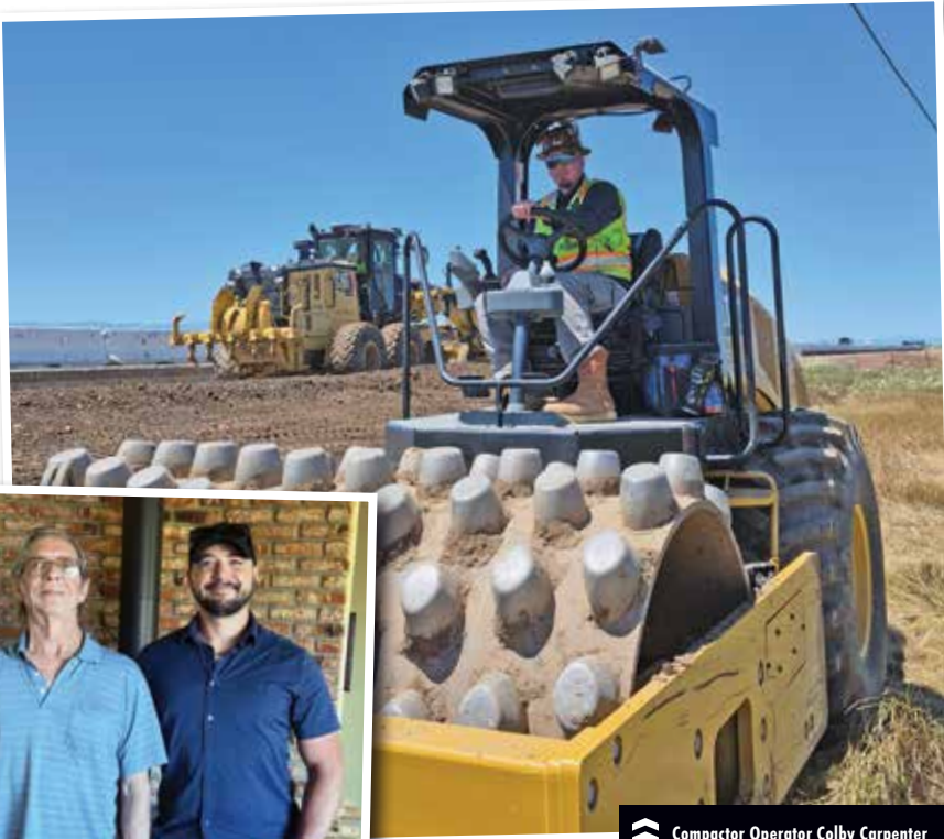
« Compactor Operator Colby Carpenter works for DeSilva Gates Construction.
