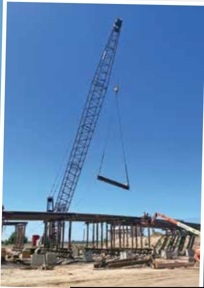
Members with Myers and Sons work on the North Corridor bridges.
