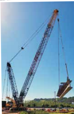
Members work on the Cordelia Truck Scales Improvement Project.
