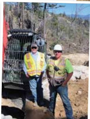
From left: Matthew Sage and Chad Pope are part of the Buckhorn Summit slide repair crew.
