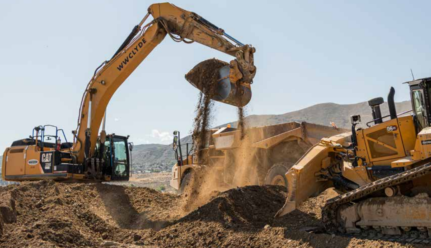
Excavator Operator Paul Koyle works for W. W. Clyde.
