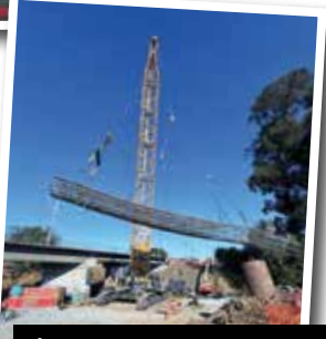
Legacy Foundation Crane Operator Gerardo Lopez trips a 4,7000-pound rebar cage.
