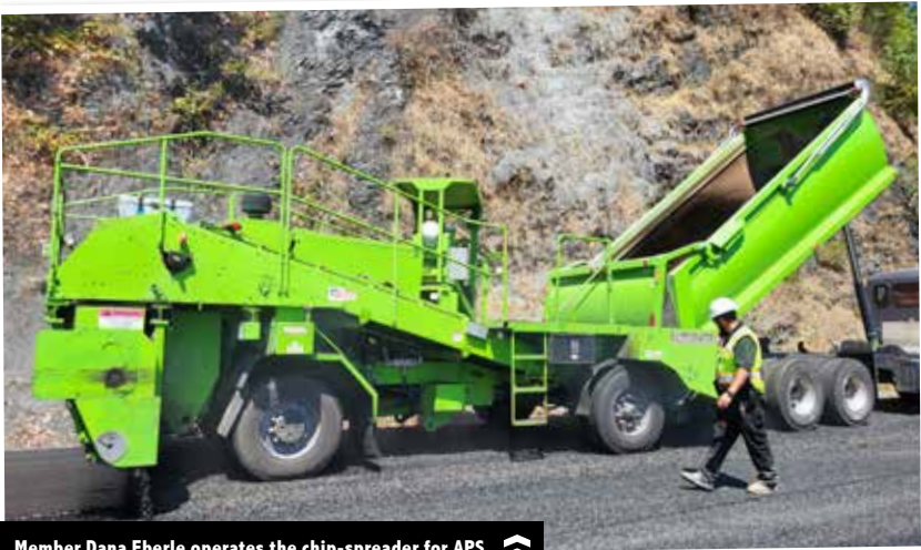
Member Dana Eberle operates the chip-spreader for APS.
