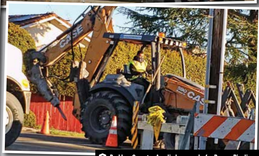
Backhoe Operator Aurelia Leon works for Ranger Pipelines.
