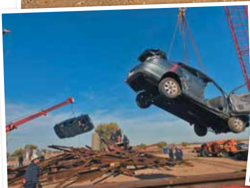
OE3 crane apprentices help create scenarios, so firefighters can practice structural collapse work.
