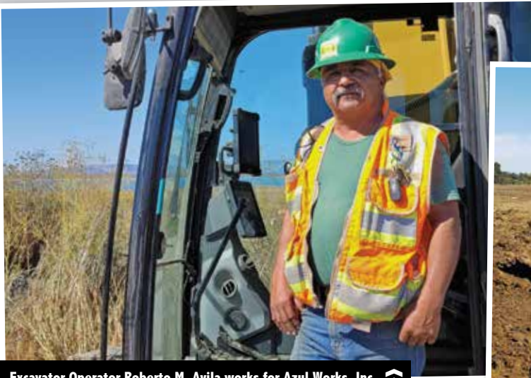
Excavator Operator Roberto M. Avila works for Azul Works, Inc.
