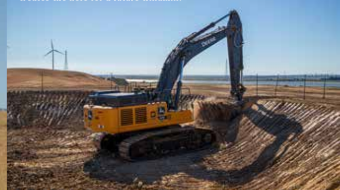
Excavator Operator Brian Vanlehn creates the hole for a future windmill.
