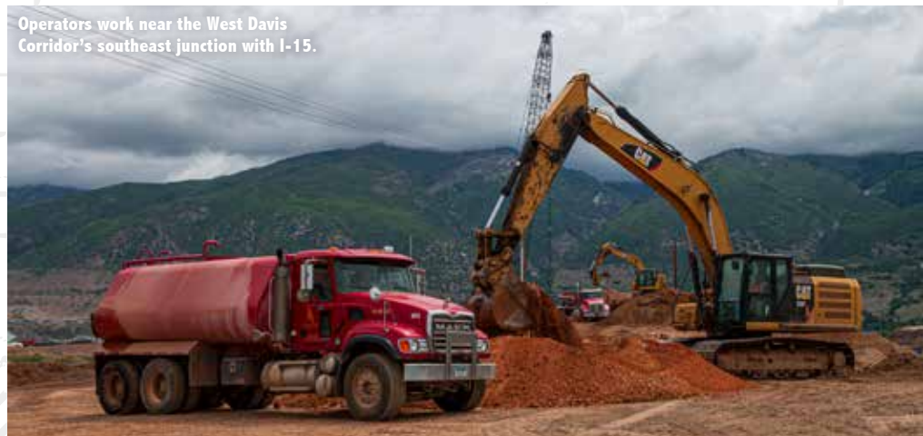
Excavator Operator John Gray.
