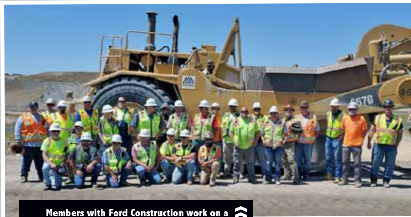
Members with Ford Construction work on a project at the Kiefer Landfill in Sloughhouse.
