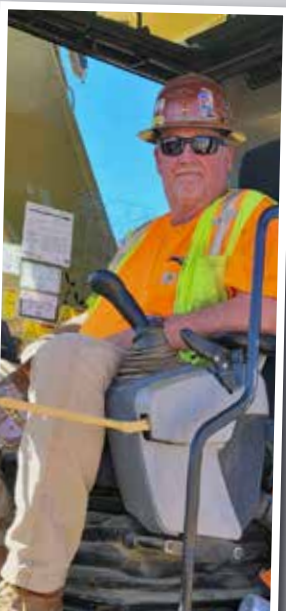
Excavator Operator Robert Kole is digging trenches for Mountain Cascade.
