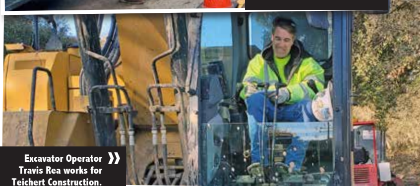
Foreman Margarito Perez performs emergency work in Blackie Road in Prunedale.
