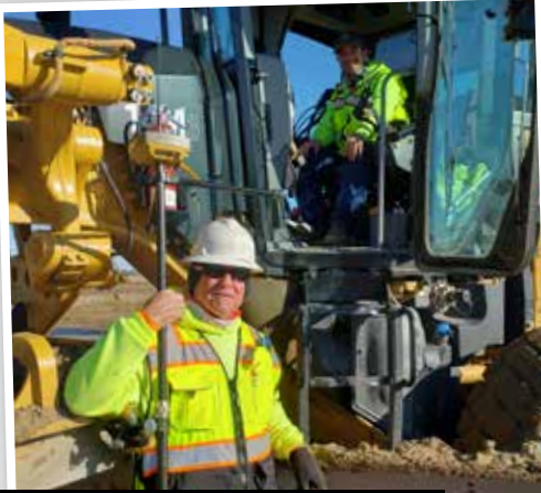
Members Chris Beutel and Simon Mattos work for Knife River Construction.
