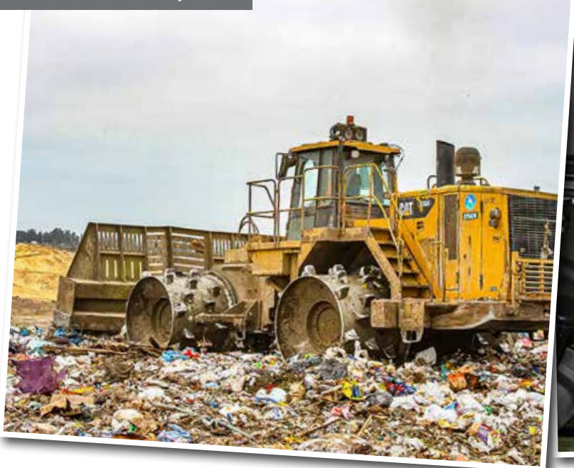
Members with MRWMD manage the landfill site in the Monterey area.
