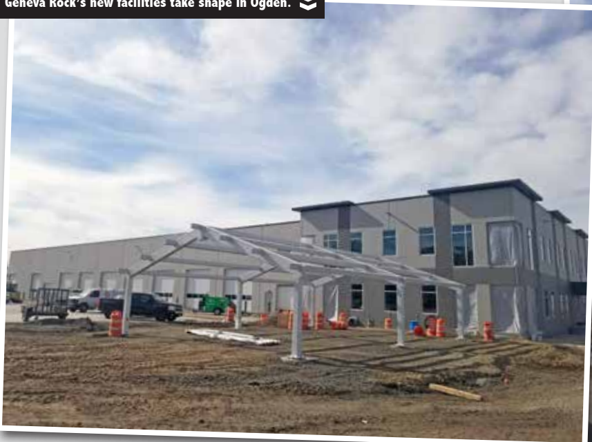
Geneva Rock's new facilities take shape in Ogden.
