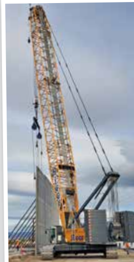
Freedom Crane Service Operator Leonard Massie and Oiler Terynn Achuleta set panels.
