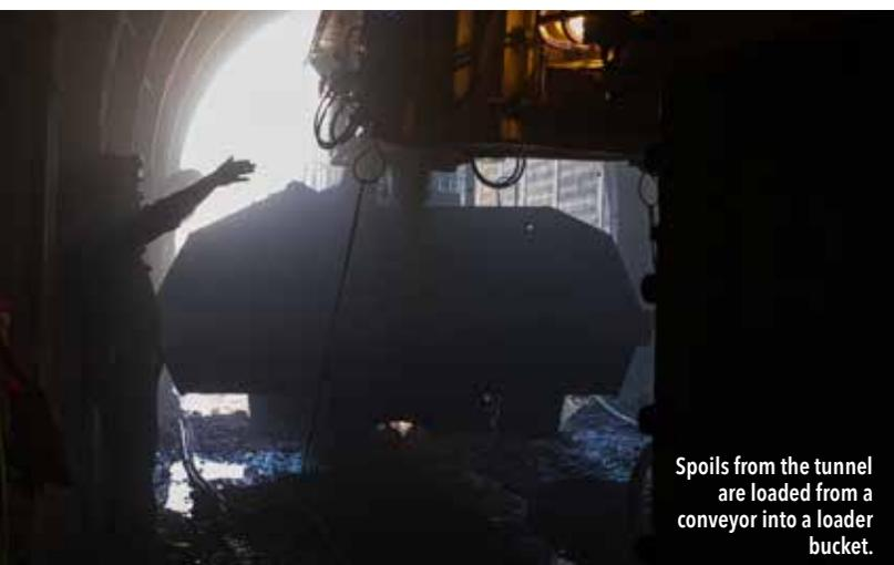
Spoils from the tunnel are loaded from a conveyor into a loader bucket.
