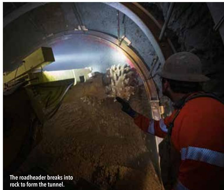
The roadheader breaks into rock to form the tunnel.
