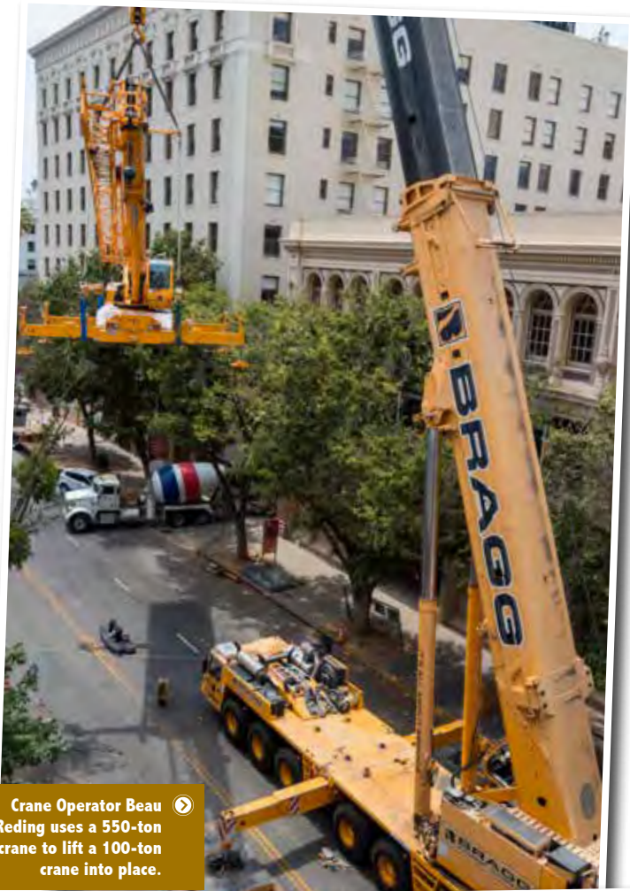
Members with Bragg Crane place a 100-ton crane on the roof of a building in downtown Sacramento.
