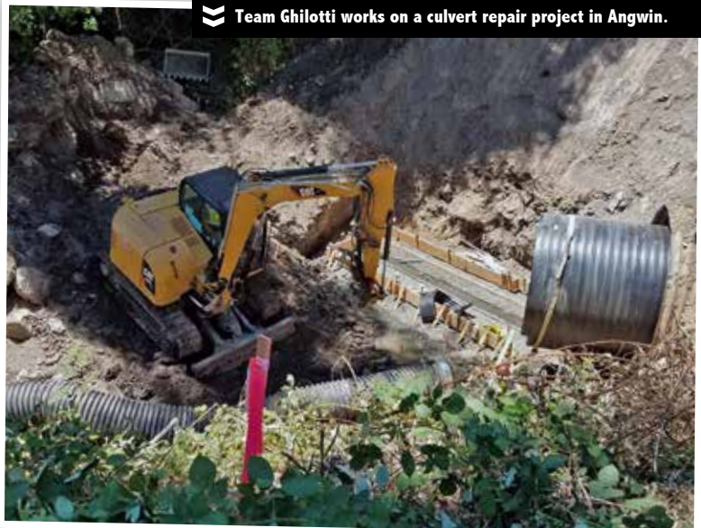
Team Ghilotti works on a culvert repair project in Angwin.
