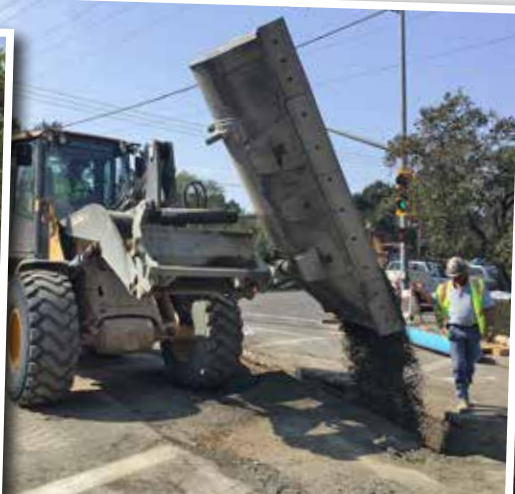
Foreman Tommy Palmer Jr. (above and right) signals Loader Operator James Huppert.
