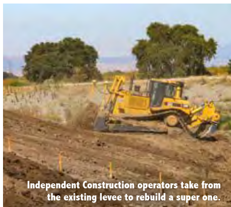
Dozer operators push scrapers, as they collect material for the super levee.
