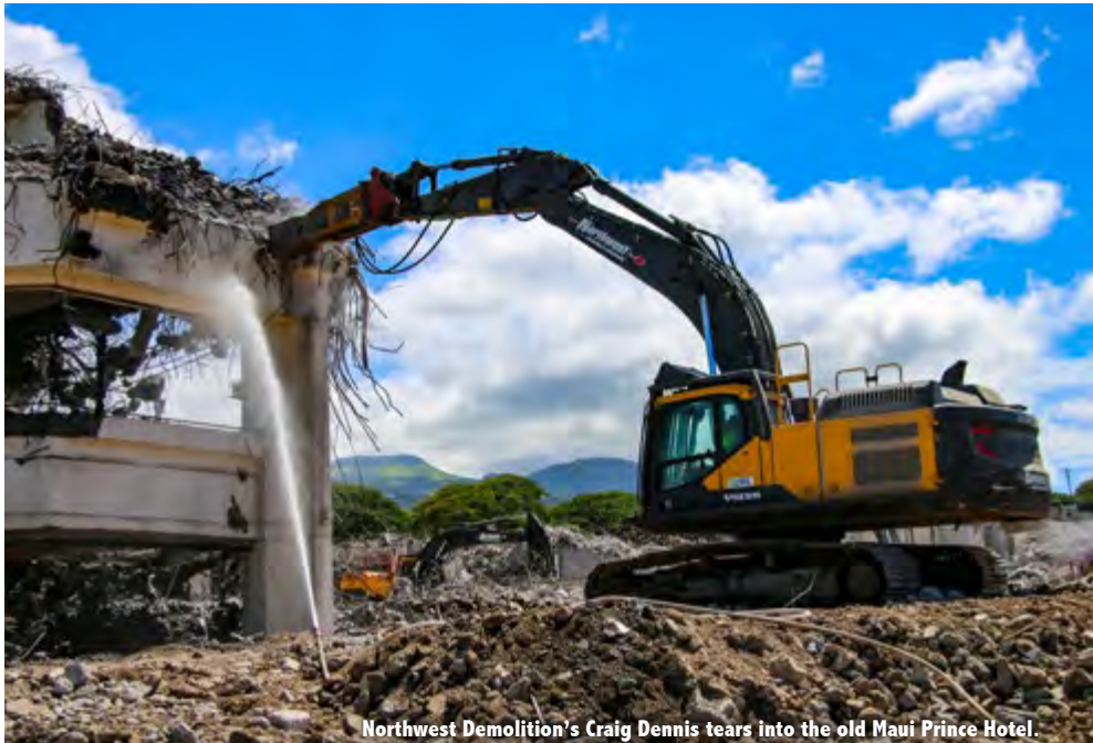
Northwest Demolition's Craig Dennis tears into the old Maui Prince Hotel.
