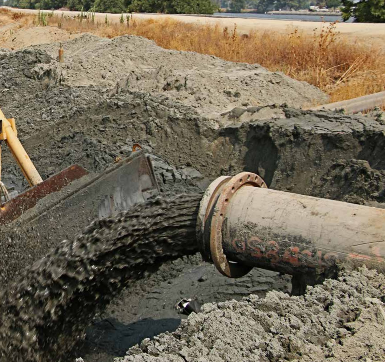
Dozer Operator Dan “Hambone” Authier deals with the spoils from the Port of Stockton’s San Joaquin River. See more of his work with Ross Island Sand and Gravel company’s giant 3,000-horsepower cutter suction dredge on pages 18-19. The spoils from the pipe in this photo are suctioned using Ross Island’s Dredge No. 8.
