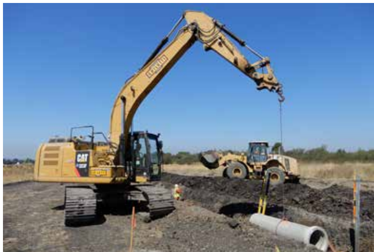
Excavator Operator Wylee Buck lays pipe for a housing project in Rohnert Park.
