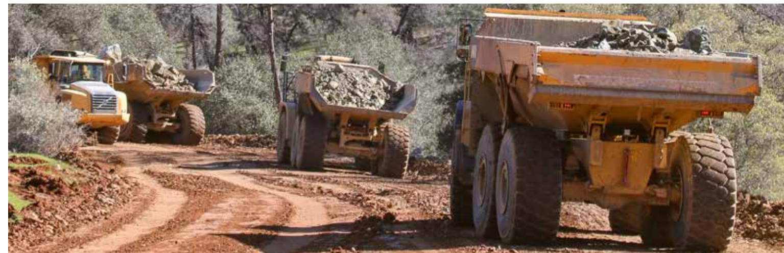
The $275 million Oroville Dam replacement project continues to provide huge work hours for District 60.
