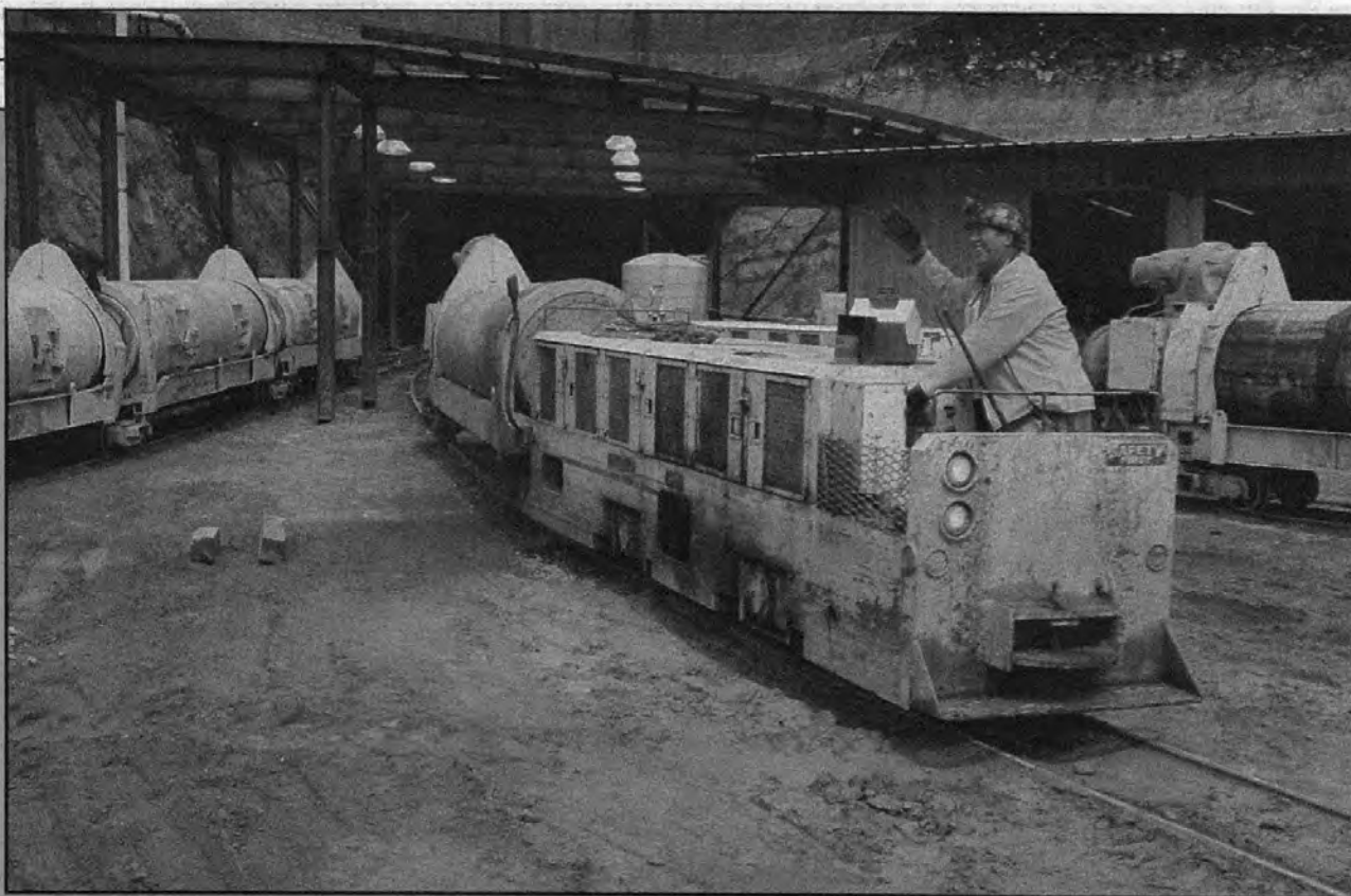
Loaded up with fresh concrete, a Local 3 member drives his muck train back into the tunnel.
