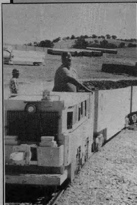
Below: Locomotive Operator Kenneth Walters brings out material from inside the tunnel.
