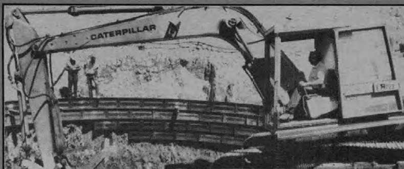
Above: Hydraulic Excavator Operator Paul Holt digging the 20-foot diameter steel and concrete reinforced water inlet.
