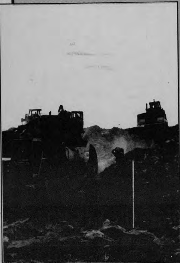
Above: "Catskinners" are leveling this 70-foot hill, which is full of rock, and moving the material to a flat area on the other side of the subdivision (below).
