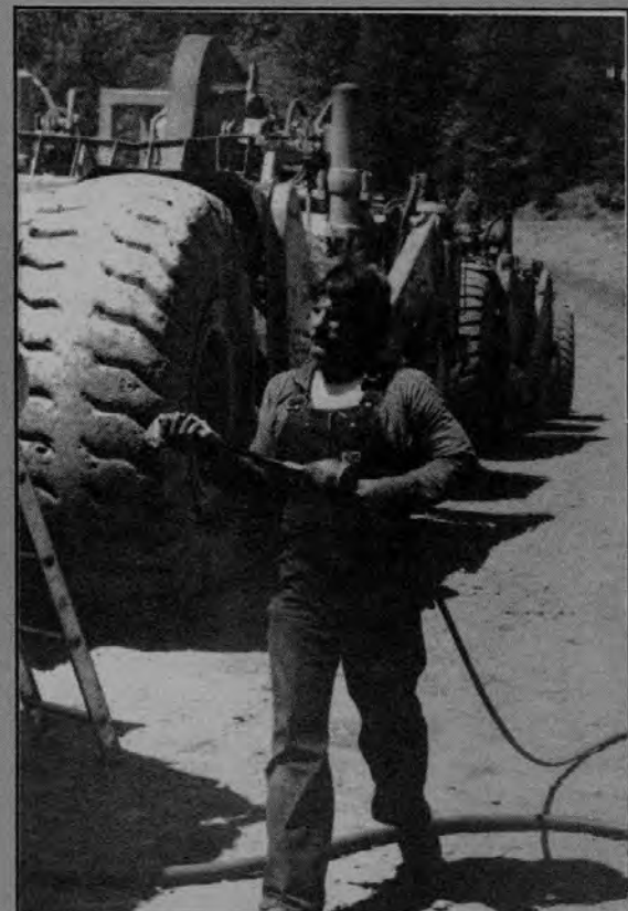
While the operators break for lunch, the lubemen move in to perform some preventative maintenance. Apprentice Lubeman Mike Gills (right) readies his lube gun, while Journeyman Lubeman Don Campbell (left) lubes a 631 scraper at the Shotgun Creek Project.
