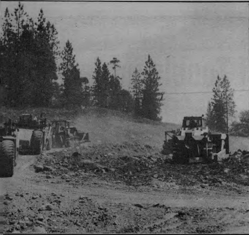
At the Shotgun Creek Project, eight 631 scrapers are working double shifts moving 6,000 yards of "tough muck" a day from a cut (left) to fill (right).
