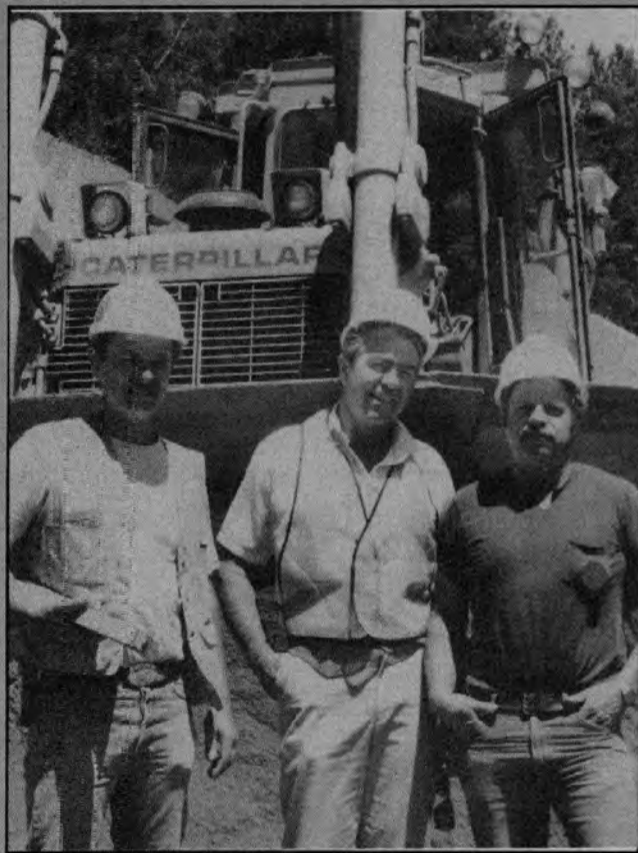
From left to right: Grade Setter Terry Porter, Local 3 Business Agent Wendell King and Dozer Operator Art Fodge at the Slate Creek Pro- ject.
