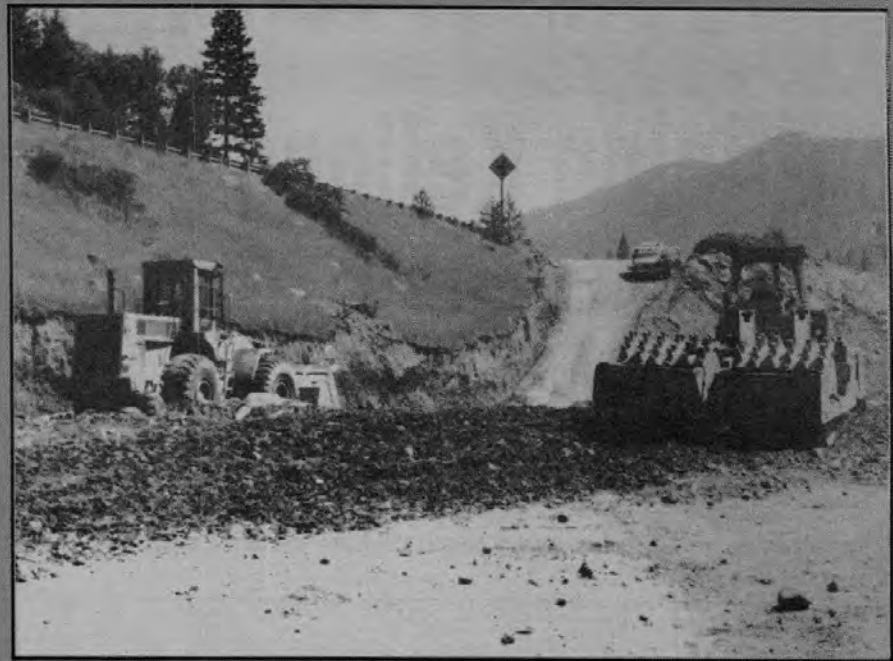
At the Shotgun Creek Project, eight 631 scrapers are working double shifts moving 6,000 yards of "tough muck" a day from a cut (left) to fill (right).
