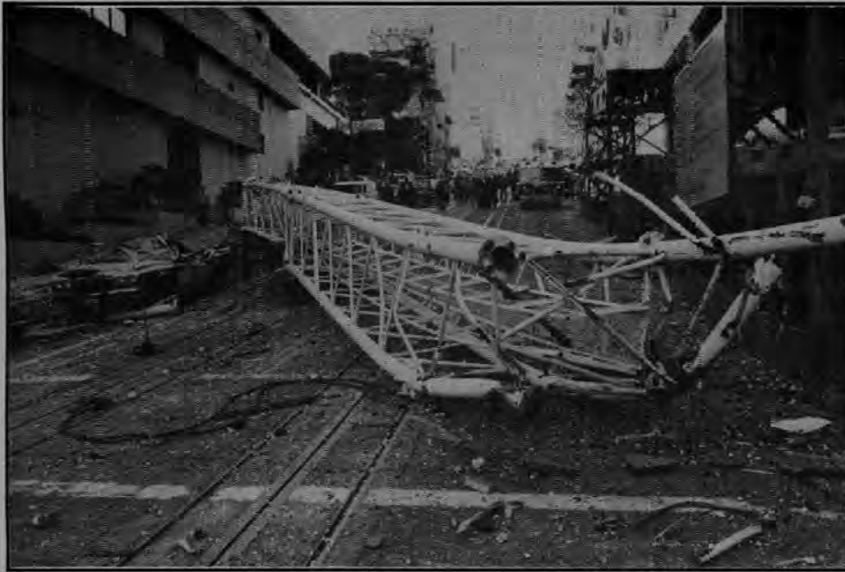
The backward force of the crane caused one of the tower's vertical members to snap. Part of the crane's boom (above) came to rest on California Street. Three passengers in the car at left were injured, as were 19 others on the ground.
