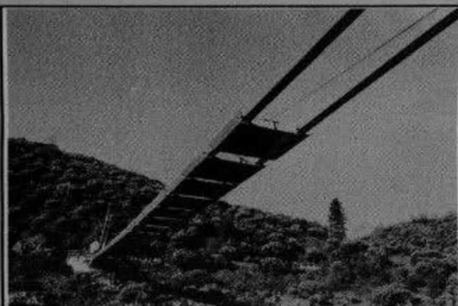
Segments were pulled out on cables then trued and plumbed.
