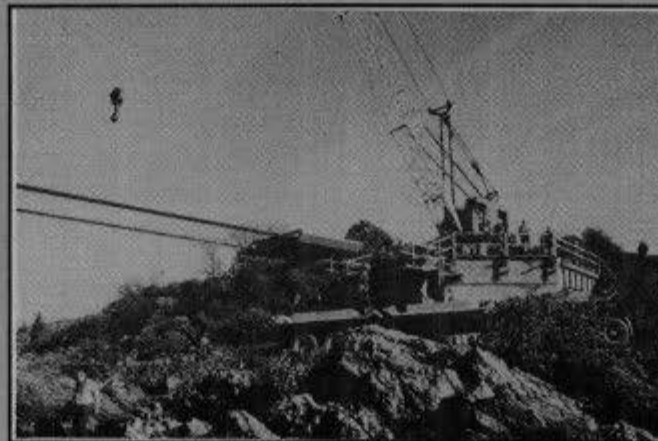
A crane was used to hoist segments into place.
