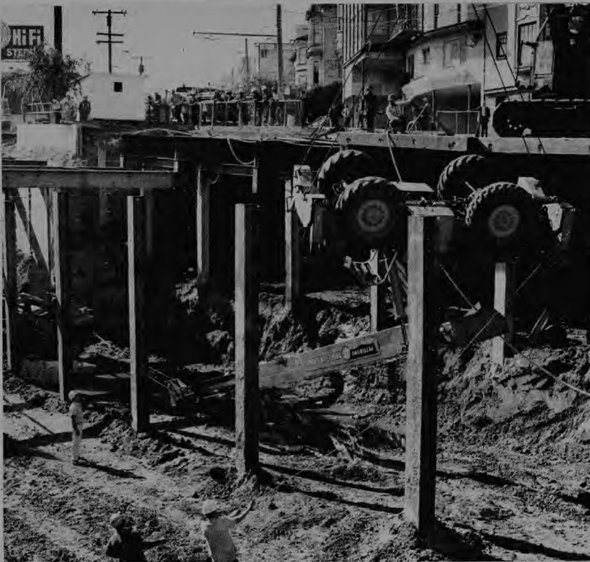
OPERATING ENGINEERS pull a self-propelled boom-type lifting device out of the excavation of the San Francisco Municipal
