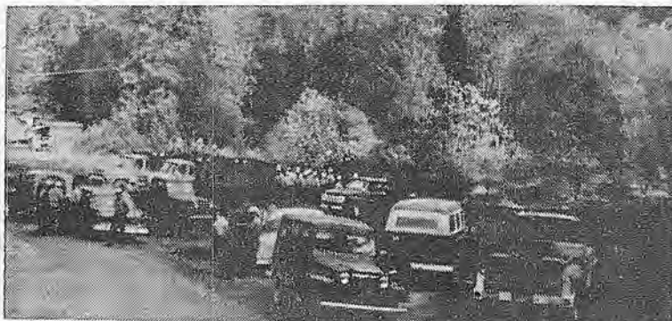
FIRE SEASON is still on in the north-state timber country, and Engineers are often key men when fires occur. This view shows firefighters after a job "well done" near Willits.
