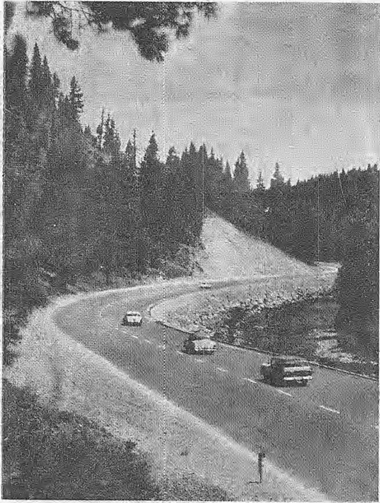
SIERRA HIGHWAY PROGRAM —Nearly $100 million in highway contracts are underway or set to go on mountain highways at the present time, a program designed to get these vital routes in shape for the steadily increasing population load, plus this winter's Olympic Games at Squaw Valley. Major jobs are set on Highways 40, 40A, 50, 49, 99, 20, and 89. Above view shows new road on State Route 89 in Placer County near Cabin Creek, 2 miles south of Donner Creek underpass.
