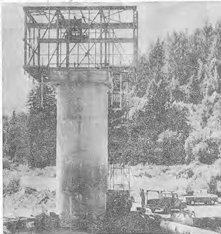
WHAT IT IS? This odd-looking tower is one of two huge wells in the bed of the Russian River near Wohler's Bridge in the Forestville area. The wells sink 80 feet into the ground and will supply 44 million gallons of water a day for the Sonoma county area. Framework at top is to hold three 1,000 horsepower pumps. Wells are part of a $12 million water development project.
