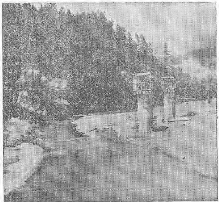
Here's another view of the two wells in Russian River near Forestville that will supply 44 million gallons daily for Sonoma county.
