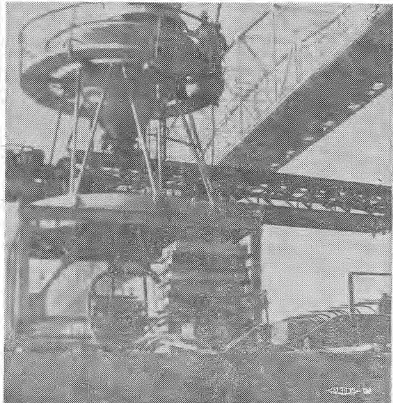
This view shows concreting work on the top of Pier No. 2 on the new Carquinez bridge. Material is dropped from the circular bin to the travelling belt below.
