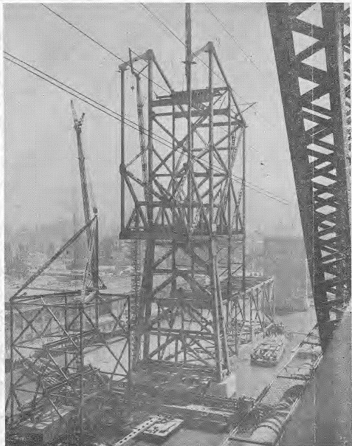
CARQUINEZ TWIN —Work is moving fast on the big twin-bridge job over Carquinez Straits. This view shows American Bridge Company's derrick and two traveler cranes on erection of
