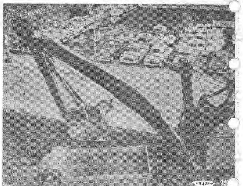
MONSTER IN THE STREETS. —That's what this long boom backhoe Northwest 80 looks like with the toy automobiles behind it. It is the Rados storm drain job on Carson-Cabrillo Ave., Torrance, Bro. E. W. Traver, operator, and Bob Welch, oiler. (Photo by J. M. Gatewood.)
