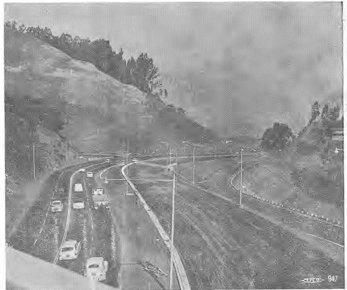
Work is rapidly drawing to a close on the mammoth Waldo grade approach to Golden Gate Bridge, which at the time it was awarded was the largest single highway contract ever made by the state. It includes several giant fills, bridges, underpasses, and a twin to the existing tunnel. Opening of the tunnel took place on Sept. 19. This is an Atkinson job. Double-track on the northern highway outlet for
