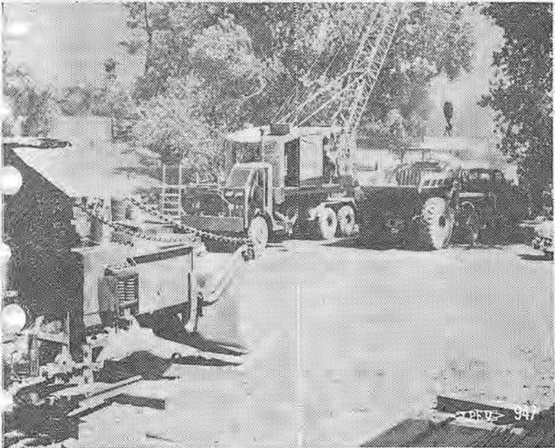
HEFTY TUNNEL JOB —There's a 34,000-foot hole in the ground being dug on the big Feather Poe power project by Operating Engineers and it is keeping the tunnel stiffs well occupied. The 24-foot shaft will cost $15 million and last 30 months. This picture shows Utah-Bates, Rogers yard at Oroville where Poe job equipment is repaired, received, and shipped out. Included is a 25-ton Koehring crane with Bro. Tommy Kennedy, as the operator and D. J. Elston, "newly married man," as oiler. Also shown is a Conway 100 mucker.
