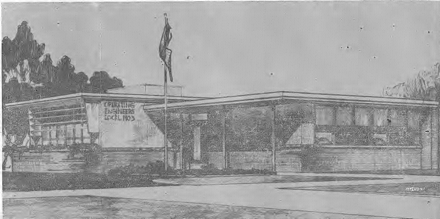
What So Proudly We Hailed—Operating Engineers Local Union No. 3's New Home in Marysville
