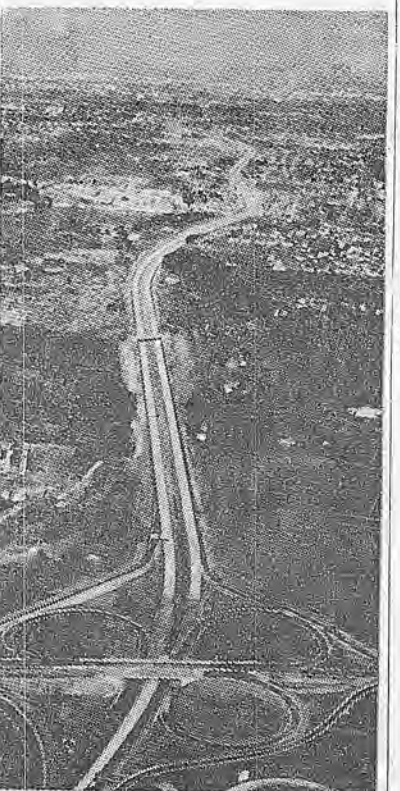
LOS GATOS Freeway — new sign Route 17 from Route 42 in Los Gatos to Bascom Ave., is now opening to traffic.
