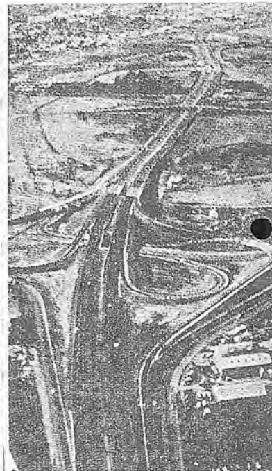
BAYSHORE - REDWOOD This shows relocation of Bayshore freeway in Redwood City, showing Harbor Blvd. interchange in foreground.
