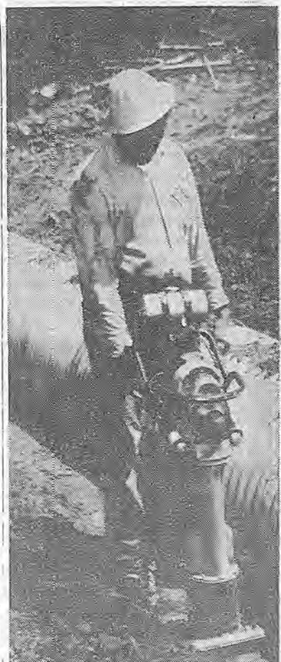
TAMPER is used on backfill around 36-inch pipeline on Trinity project road relocation, Ridgeville to Covington Mill. Ray Kizer Const. co.
