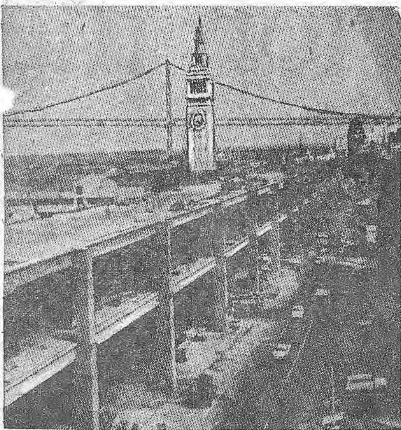
EMBARCADERO NEW LOOK —The 1.2 mile, $9½ million, double-deck freeway from the Bay Bridge to Broadway, along the waterfront, is moving fast these fine days. Southbound motorists, riding 70 feet above the street, will get a spectacular view. The job is to be completed late this year. Contractor is Chas. L. Harney.
