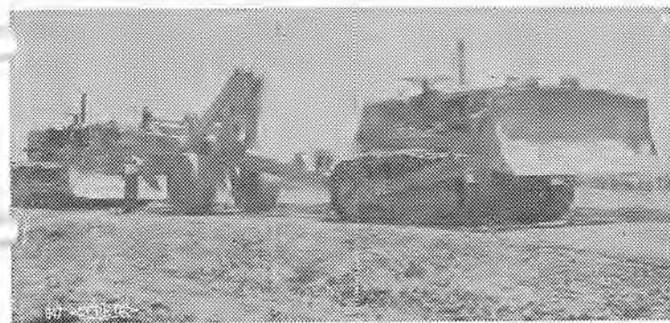
GIANT SIZED RIPPER —This view shows Bro. Lowell Surface pushing on a D-9 and Bro. Al Tribble pulling on a D-9. This big iron is in use on the Rocky Ridge road between Folsom and Roseville, Stecker and Scott, contractors.
