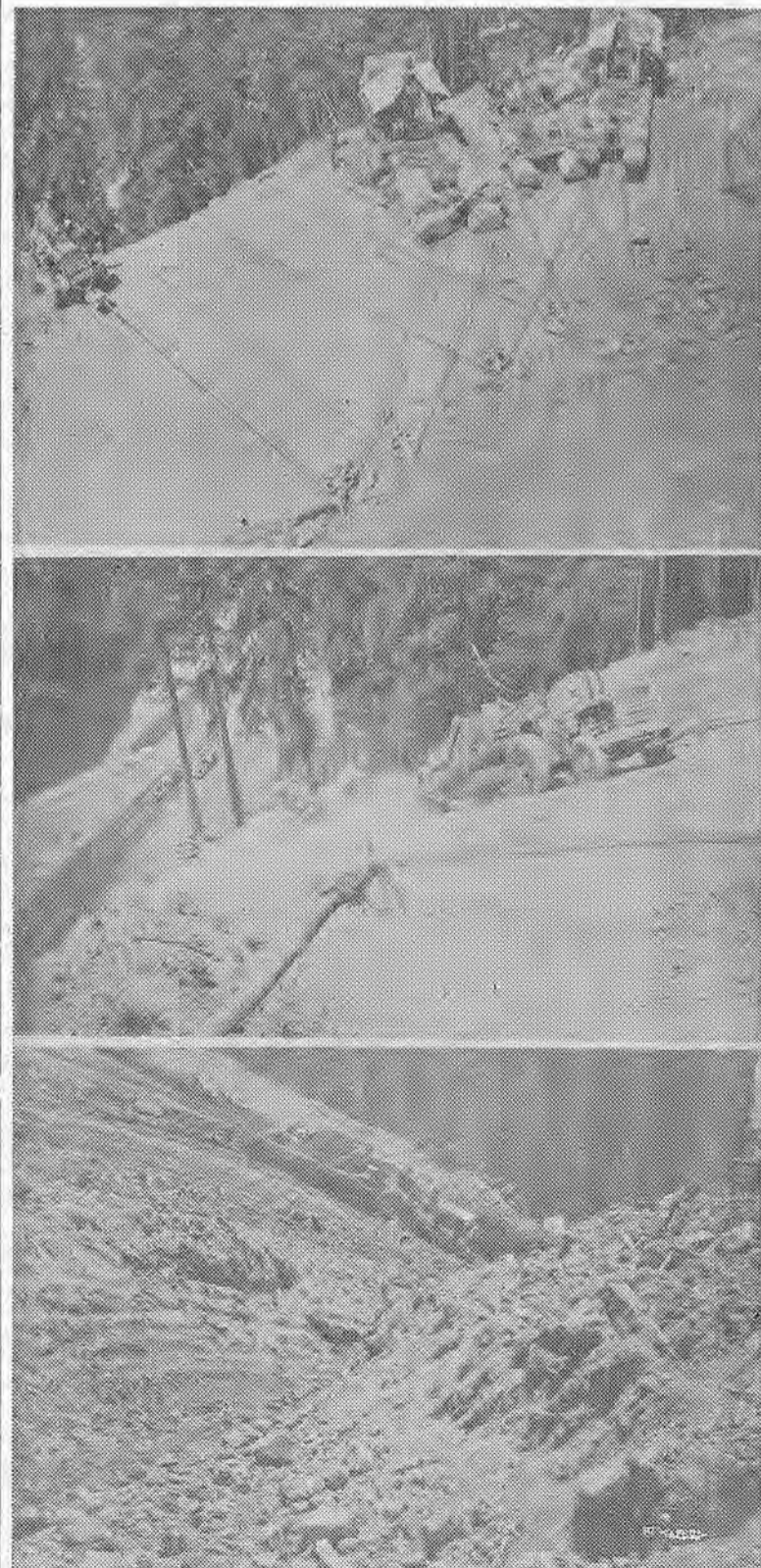
These views show a DW-20 on its way up the hill at the big cut on Highway 101 at Dyerville, and on the way down. Also shown are the three of the four donkies used to pull the rig up the slope. Guy F. Atkinson Co. will make a 400-foot cut at this point.
