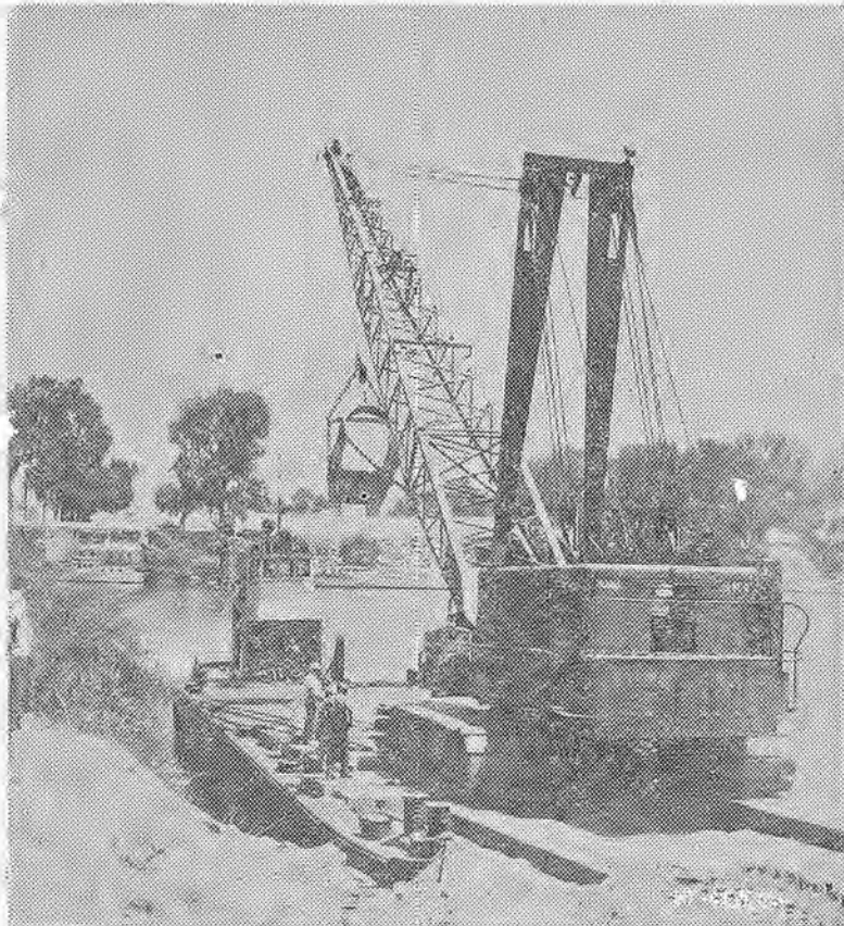
START SHIP CHANNEL —This 4500 of Luhr Brothers is being loaded on barge at Sacramento for a trip to Little Holland Island to start digging the toe drain on Sacramento's much-publicized deep water ship channel.
