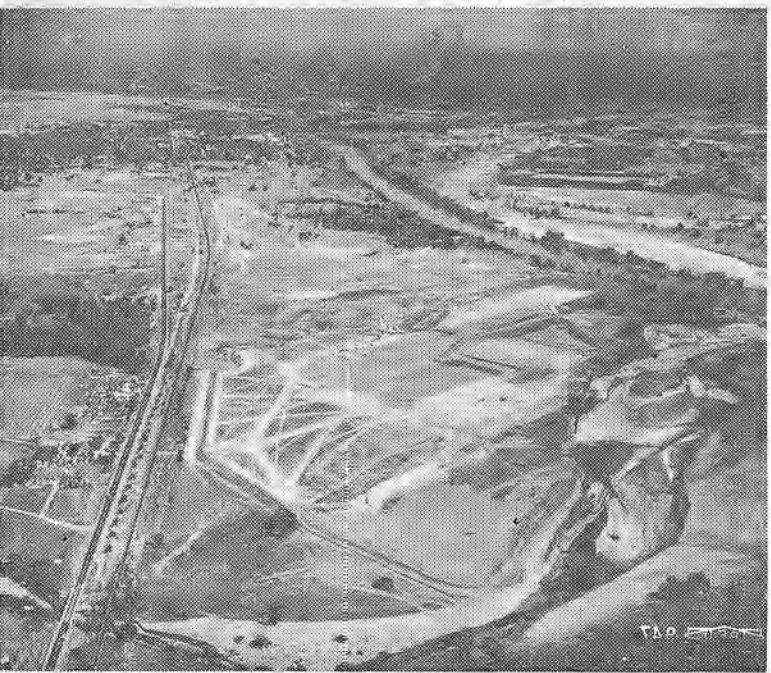
SHASTA INDUSTRY BOOM —With the $120 million Trinity power job under way, new housing, and industry, and now the $21 million Diamond Match plant under way, the north inland empire is booming. This view shows present work on the Integrated Forest Products plant of Diamond Match about two miles south of Red Bluff, off Highway 99, with the Sacramento river in background and highway at left. Del E. Webb Const. Co. and Southwest Engineering Co. are the builders.
