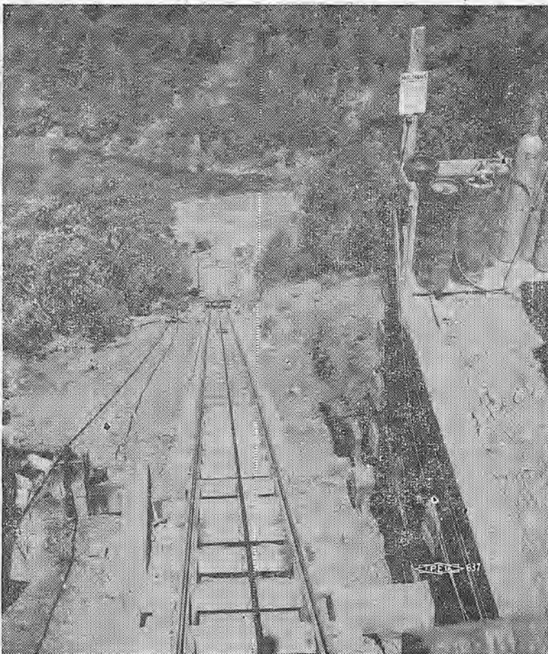
MEN VS. MOUNTAINS —Up in the Feather River Canyon a small army of skilled workmen is fighting the elements, insurmountable slopes, and mountains of granite to hew out new sources of power for growing California. This view shows a 700-foot 70-percent grade incline hoist on the Utah, Bates & Rogers Const. Co. Surge Chamber job on the PG&E Poe Power Project. Note size of auto at bottom. Operating engineer Geo. Harrison is hoist operator. (Pic by Jim Jennings and Les Collett.)
