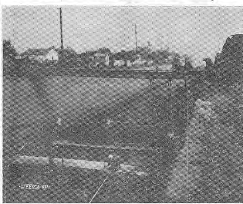
AUTOMATION IN DITCH DIGGING —Well, it had to come. It has hit about everything else, so why not the back-breaking job of ditch work. This special-built 55-foot, self-propelled concrete spreader mounted on driving wheels includes a 1½-yard cement bucket traveling across channel under control. In bottom is a special self-propelled finishing machine with vibratory screed built in. It is built up to pass over reinforcing steel and runs on headers. Location is an Army flood control job in Southern California.
