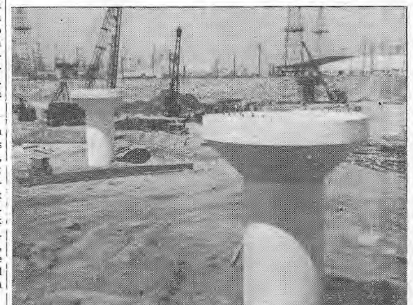
GIANT TOADSTOOLS is what these large concrete railroad bridge piers look like. They have 220 yards of concrete in them and will hold 55-ton girders on which railroad tracks will be placed. Location is 7 1/2 street across L.A. river in Long Beach.
