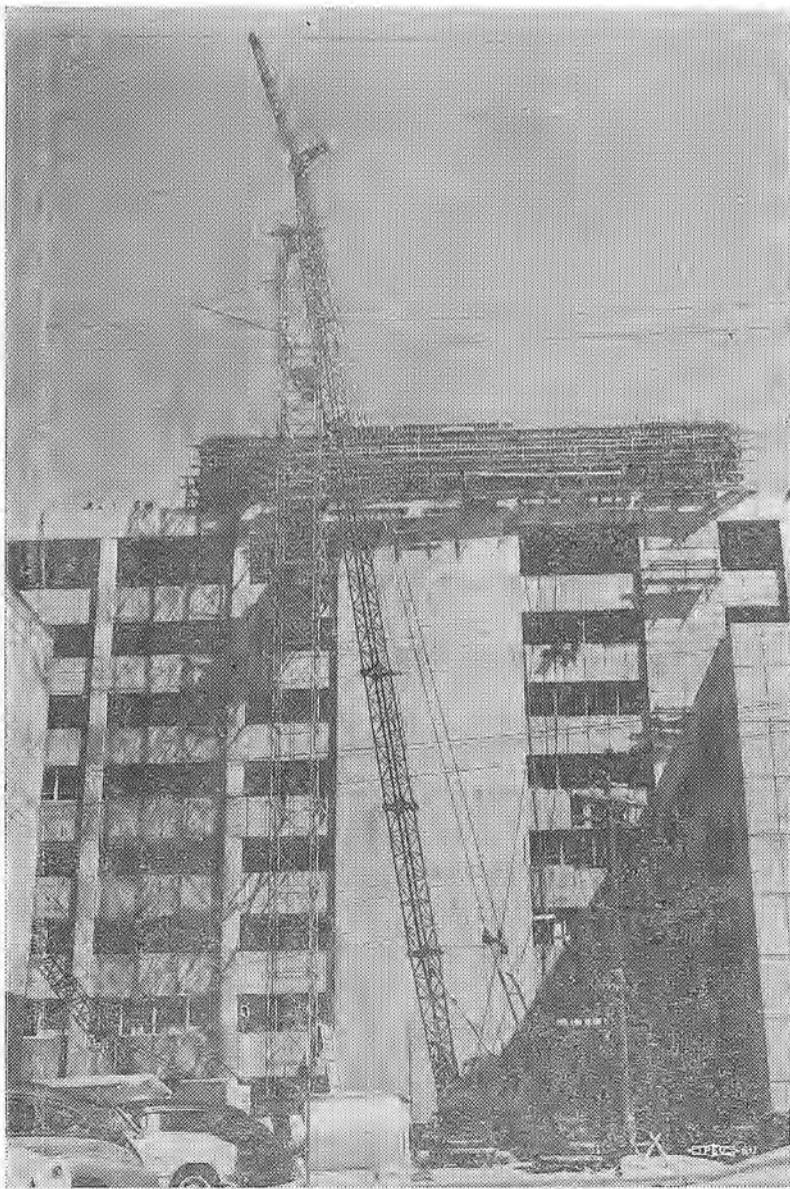
UNIV. OF CAL. EDUCATED SKY-HOOK—Shown in the picture is Datzell Rigging Company's 30-ton P. & H. Crane, with 180 feet of boom, which was used to set the stack down through the interior of the California State Health Building at Shattuck and Berkeley Way, Berkeley. Brother Ben James is operating this rig with Brother Bob Alter doing the oiling. (Picture by Bro. Jim Jennings.)
