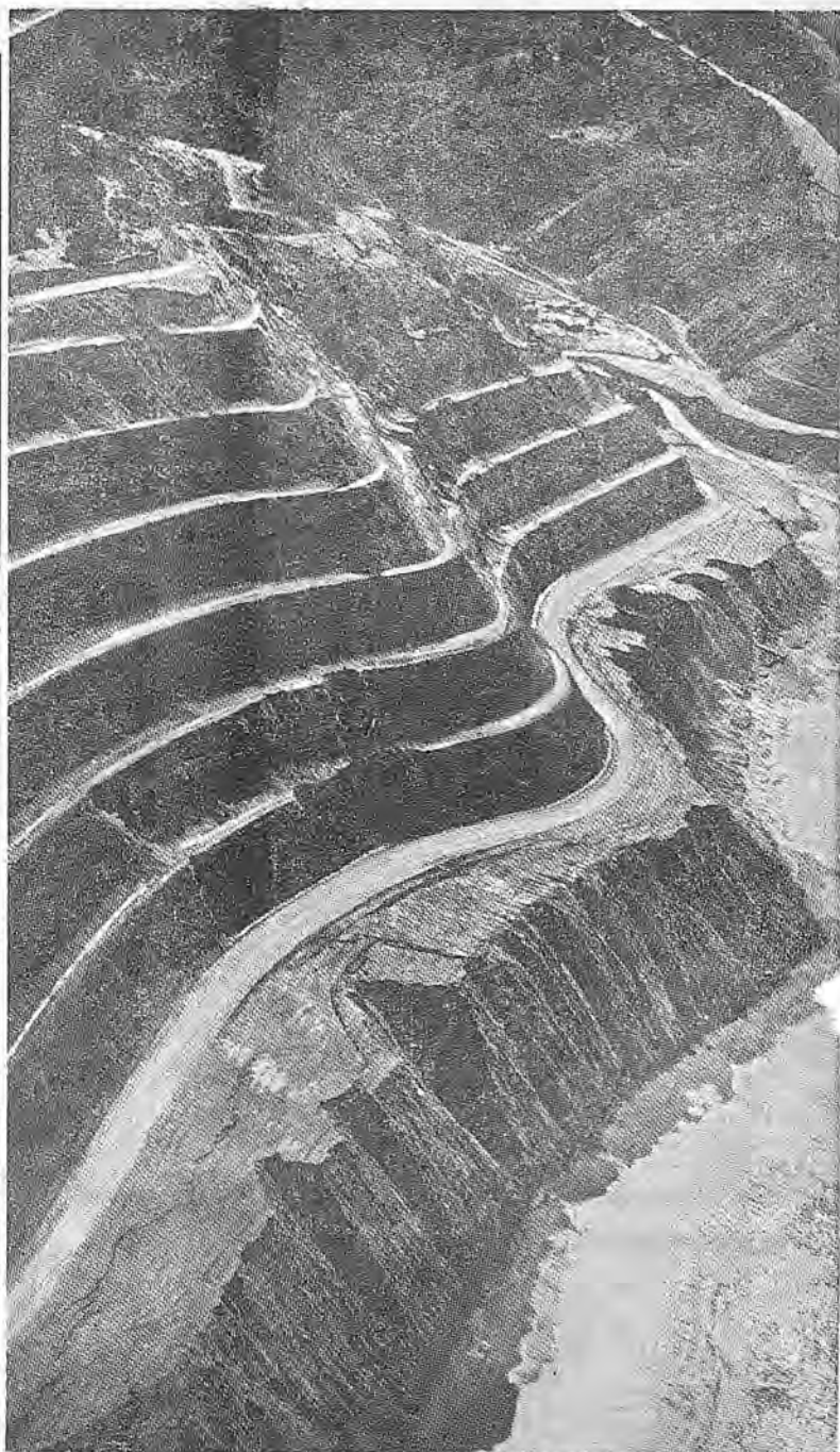
PACIFIC AMPHITHEATER—Not the rice fields of Burma, nor the copper mines of Utah, is this scene, but rather the scenic, rugged Mendocino county coastline, where it was necessary to excavate 700,000 cubic yards on a 1000-foot bluff, in six giant benches, to get a roadbed for State Sign Route 1. This was a $350,000 job by Rockport Redwood Co. at Juan Creek Bluffs under the Federal-aid Secondary Highway program. 'Tis said the Paul Bunyan of the Redwoods comes out and sits on these benches to watch the sun set in the Pacific.
