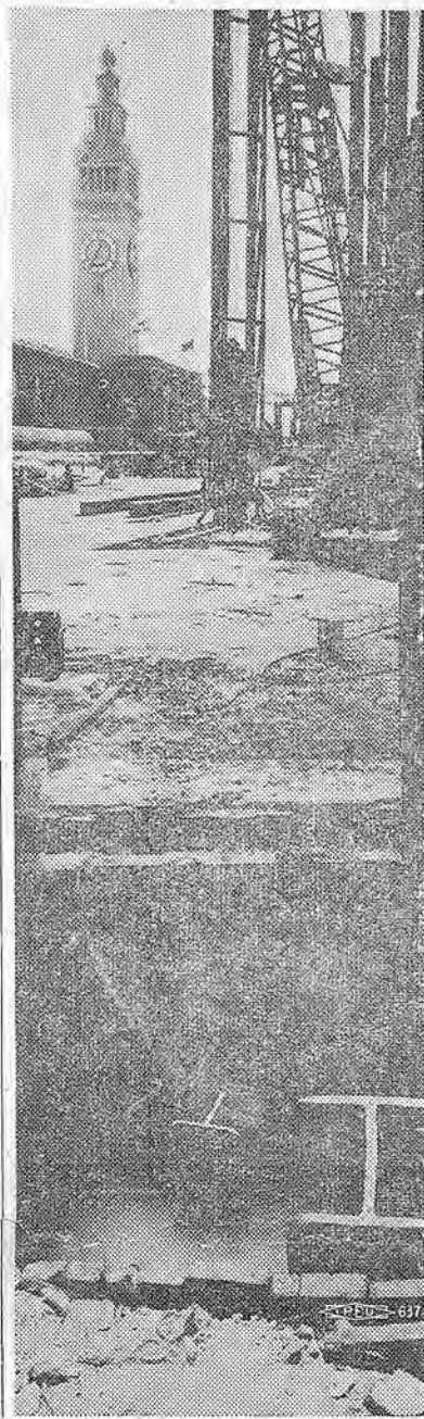
That's salt water you see in the hole cleared for driving steel piling way down into San Francisco's famed Embarcadero. The big "I" beams will give solid foundation for the two story freeway, Bay Bridge to Golden Gate, now taking shape in front of the historic Ferry building.
