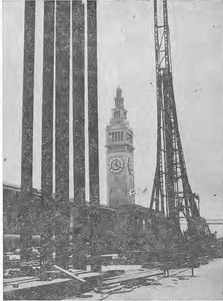
PATTERN FOR '57 along the Embarcadero these days is steel and concrete shaping up into a huge, high, fast freeway along the waterfront, bringing the era of autos right into the domain of windjammers, battlewagon, and merchantmen.
