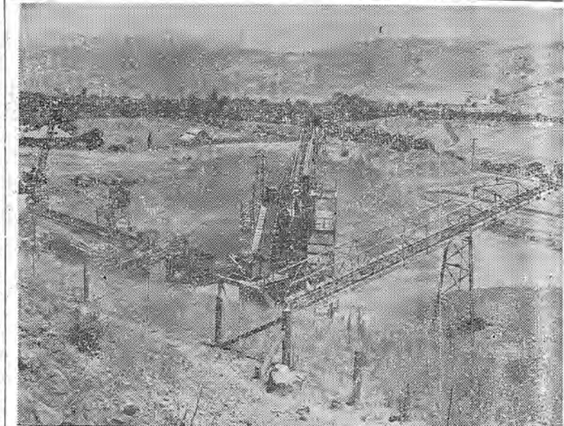
Contra Costa County's hilly interior is location for big aggregates plants. This is a view of Pacific Coast Aggregate's plant at Clayton. (Picture by Jim Jennings, Oakland office of Local 3.)
