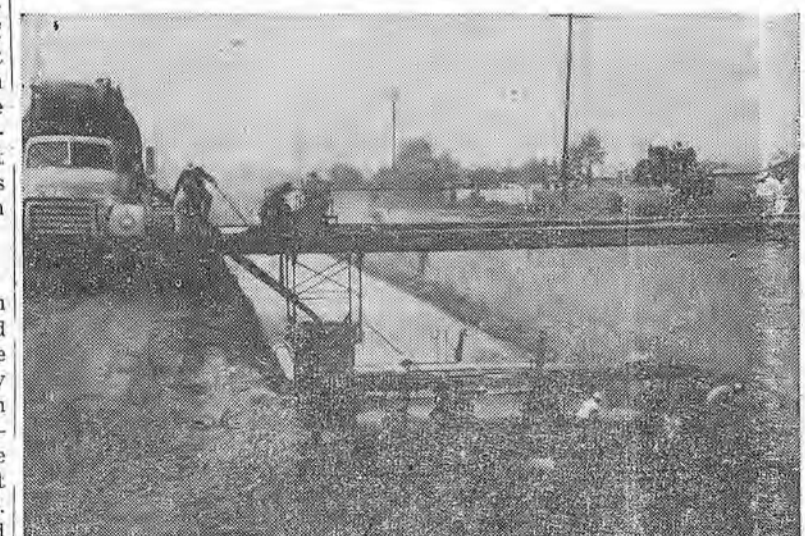
This is a front view of the Cutcrete Corp. specially built concrete spreader. The 1 1/2-yard Garbro cement bucket that travels across channel and stops where directed, is shown being filled from Transit Mix truck. Special finishing machine, passing over reinforced steel on headers, can be seen in bottom of channel.
