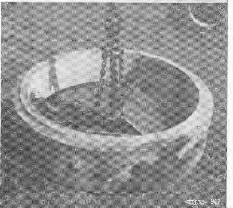
Operating Engineer Bill Holloway of Oakland, master mechanic and his assistants at the McGuire and Hester shop, have developed a cam and lever device which they call a Center Lift, which will be used in handling 30 and 40-inch manhole collars. Another example of skill and know-how by Operating Engineers. Lower picture shows the fit; upper view shows it in operation. (Pic. from Oakland office of Local 3.
