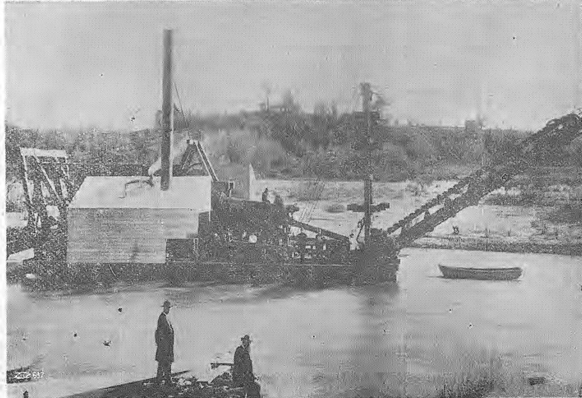
Shown above is the new and old earth-moving unit in the world, one of a fleet of seven being operated in the gold fields eight miles east of Marysville by Yuba Consolidated Gold Fields. The lower picture shows one of the first gold dredges operated in the California gold fields. It was built by the Risdon Iron Works in San Francisco in 1902. Photos, courtesy of Yuba Consolidated Gold Fields.
