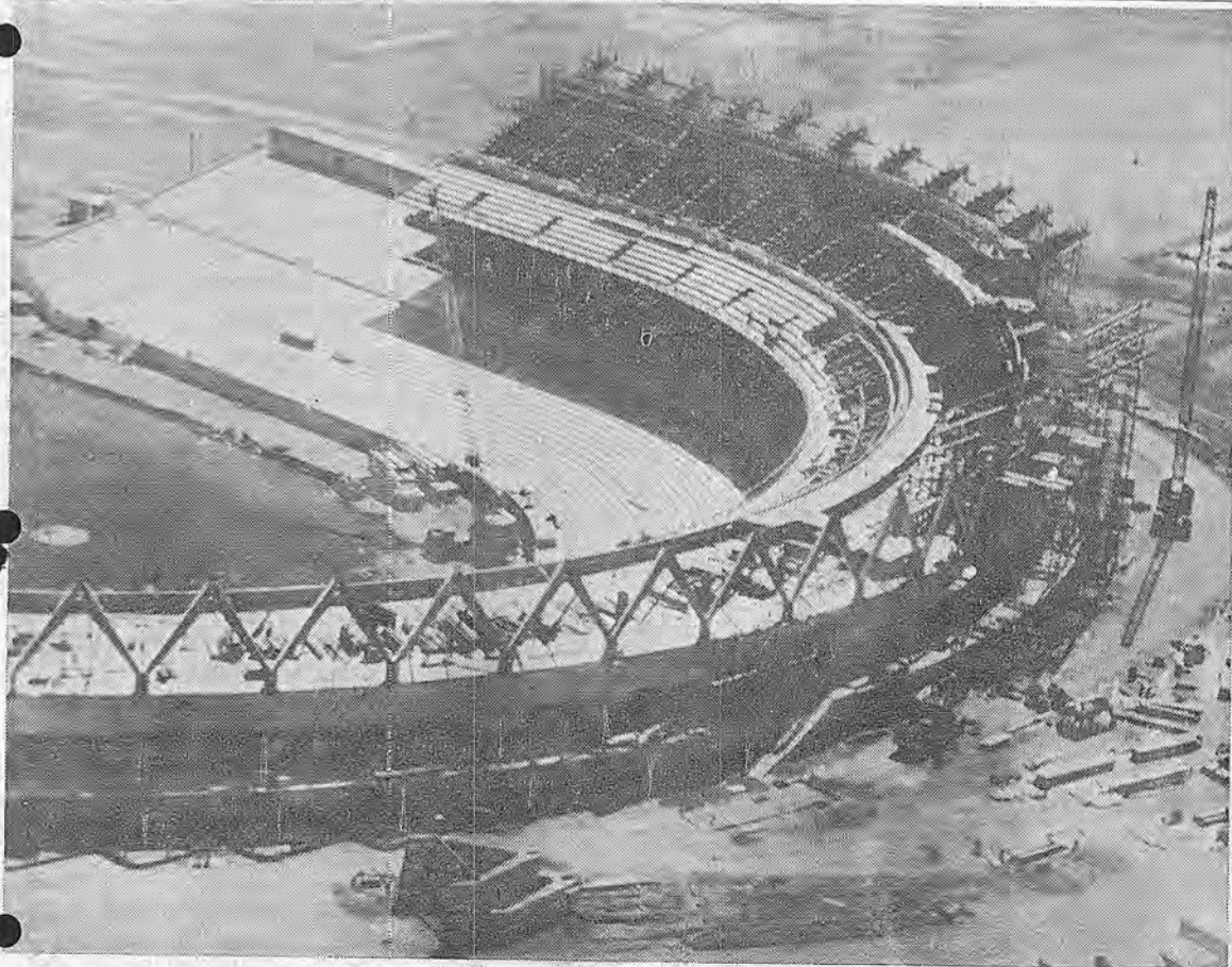
GIANT BAY BOWL —Work is pushing fast for possible fall opening of S.F. Giants' new home at Candlestick Cove. The multi-deck stadium is taking shape with help of long-leg motor cranes. That's green grass growing already on the field. For another picture of general location of the ball park, see back page.
