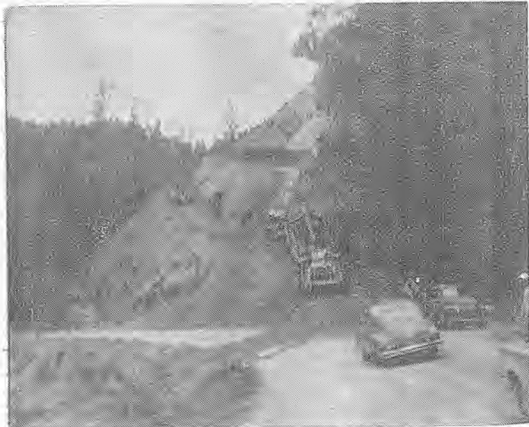
101 IMPROVEMENTS—Shown here is work progressing on the south end of the Granite job on Highway 101 just north of Willits.
