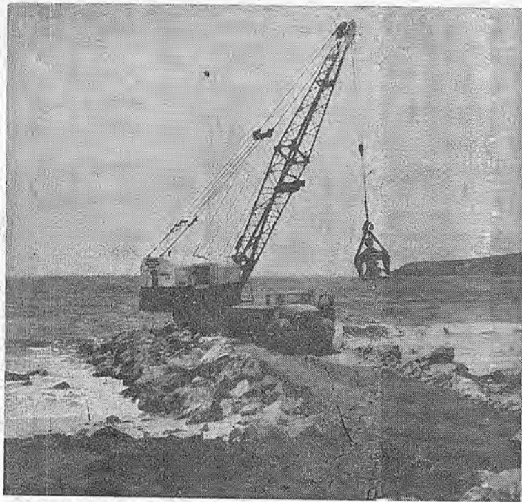
PILLAR POINT at right background will form one arm of a new harbor on San Mateo county shoreline, small boat refuge between S. F. and Monterey Bay. The other arm, an 8,000-foot rock pile is shown here taking off from the beach with Operator Orville Smith on the Granite Const. Co. rig, with son Norman as oiler. Healy-Tibbits is also in on the bid. Stone is coming from Davenport in Santa Cruz county.
