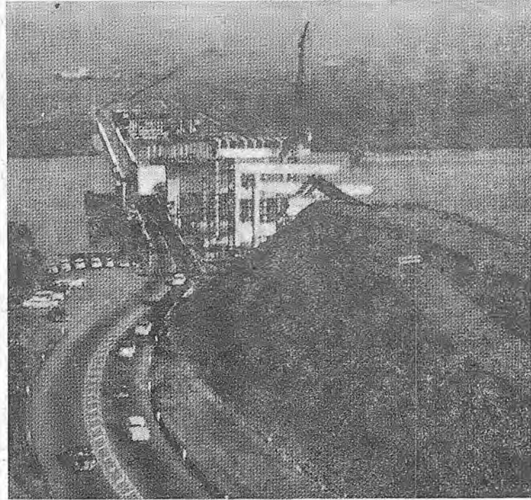
PETLUMA CREEK, historic waterway, gets a new high crossing for the highway. This view is looking east. The partially completed fill in foreground will be finished after two lanes of the new bridge are opened to traffic and the old draw-bridge is replaced.
