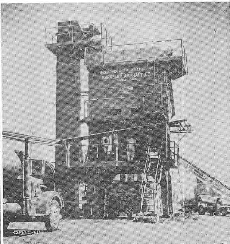
NEW HOT PLANT in Berkeley is that of Berkeley Asphalt Co. at Third and Virginia, one of the newest in the area. This view shows Bro. Harry Leonesia, boxman, loading out a truck with hot mix from the main hopper. Fireman Pete O'Neil is at left. (Picture by Jim Jennings.)
