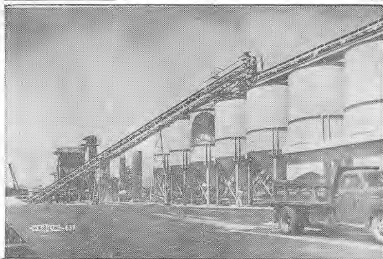
BERKELEY ASPHALT CO. is mighty proud of its brand new plant at Third and Virginia streets, Berkeley, one of the most up-to-date hot plants in this area. This is a view of the material storage tanks and conveyor belt which loads from boxcars to tanks. (Picture by Jim Jennings, Oakland office, Local 3)
